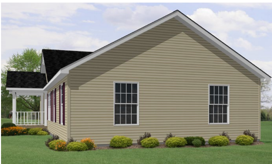
7/12 Roof Pitch with or without Attic Storage Optional Attic Window Available with Attic Storage only
