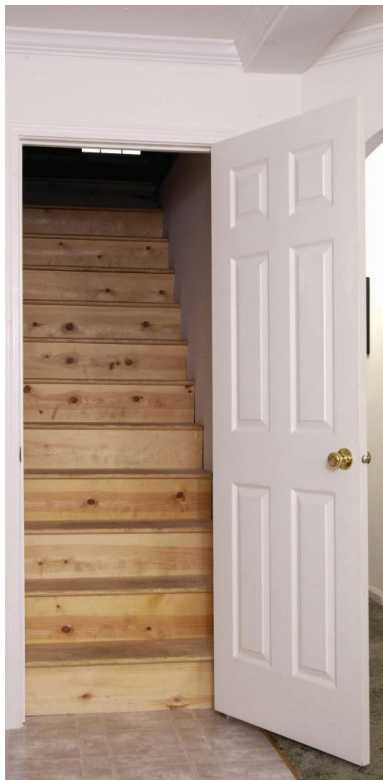
Stairwell with Light & Insulated Interior Door w/ Sweep
