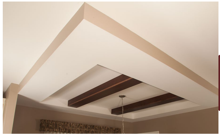
Tray Ceiling with Beams
